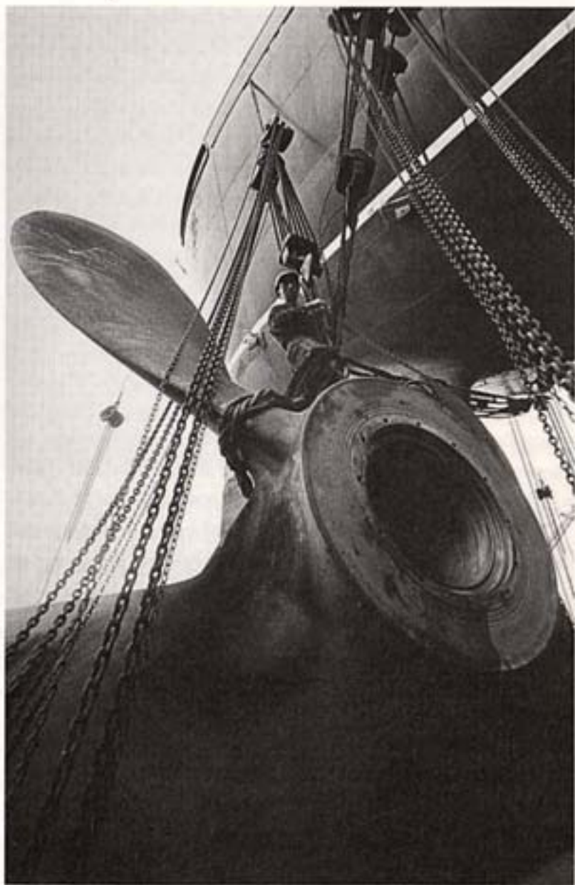
Rigging a propeller, photograph by Benedict J. Fernandez, circa 1971-1973.
