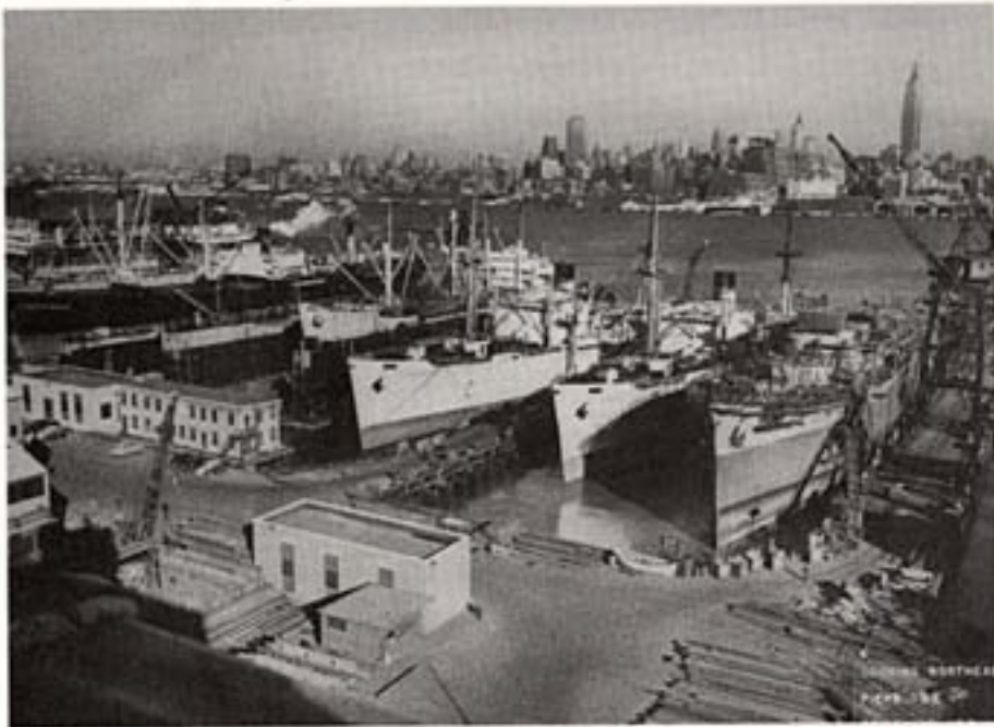
Ships in dry dock at Hoboken's Bethlehem Steel shipyard, with New York City skyline beyond, 1943.
