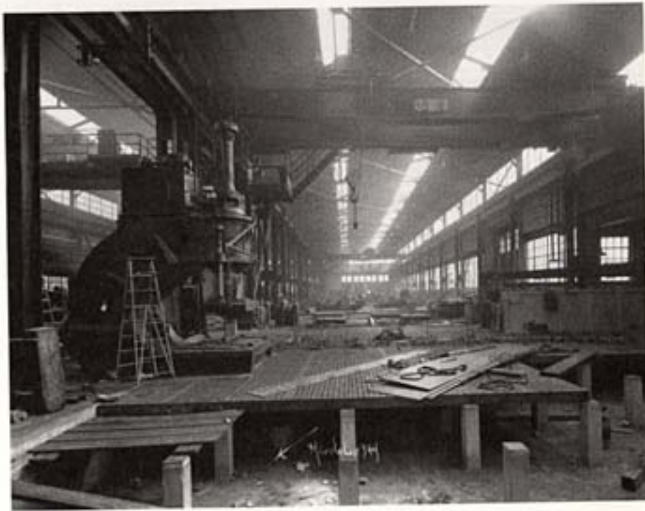
Machine Shop interior, 1944.
