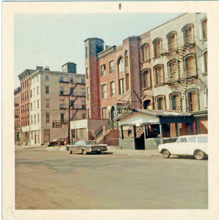
Photo of River Street, between Third and Fourth Streets, Hoboken, prior to demolition, 1969. A sign for Nelson's Marine Bar & Grill can be seen on the left; Keane's Tavern is in the center.
