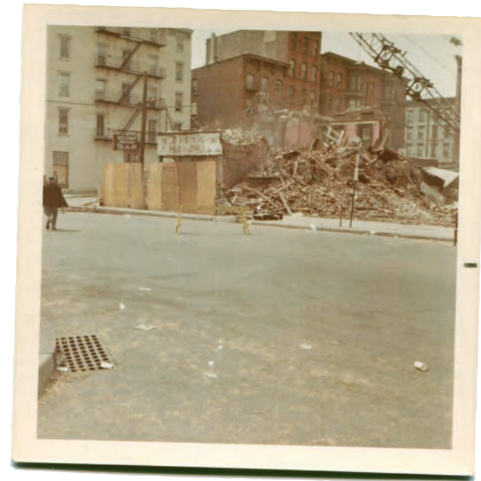
Photo of the demolition of Nelson's Marine Bar & Grill, 1969.
