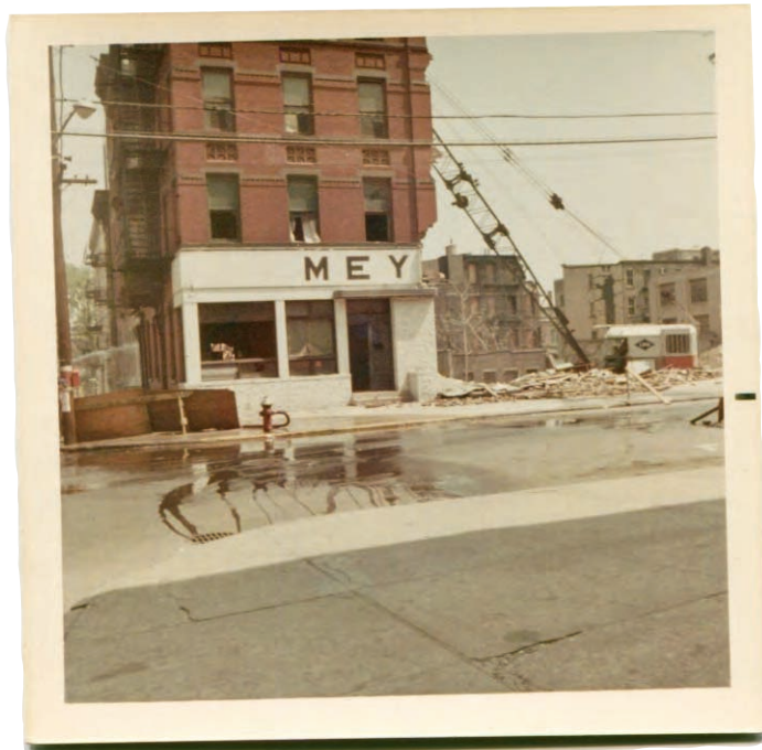
Meyer's Hotel, on the corner of Hudson and Third, was also demolished in 1969.
